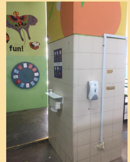
The pillar near the sink & the Basketball Court
